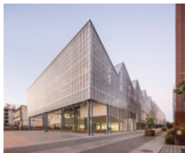
Site de Nantes. Architecture Franklin Azzi, 2017. Photo Luc Boegly
